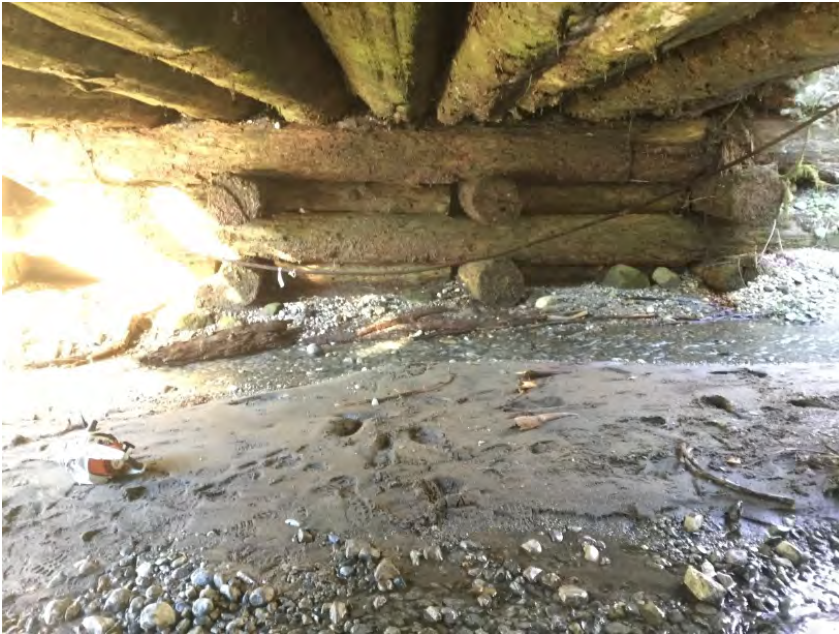
Right Bank Abutment when facing downstream
