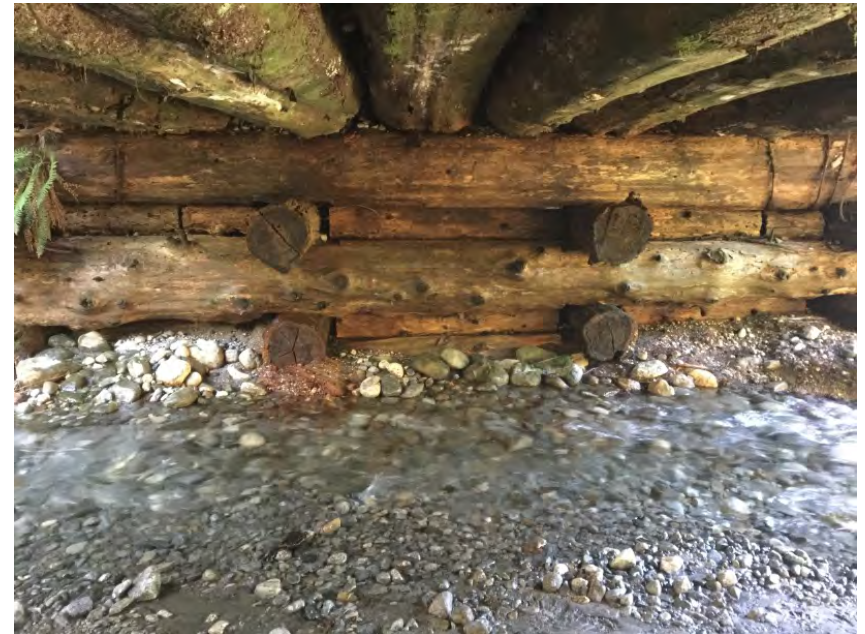
Left Bank Abutment when facing downstream
