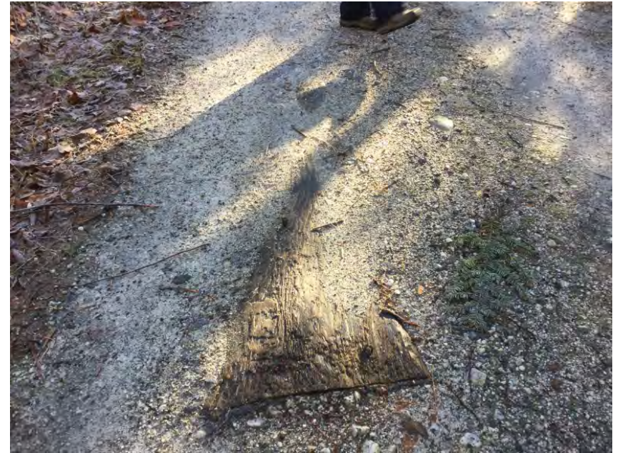
Top stringers visible from surface
